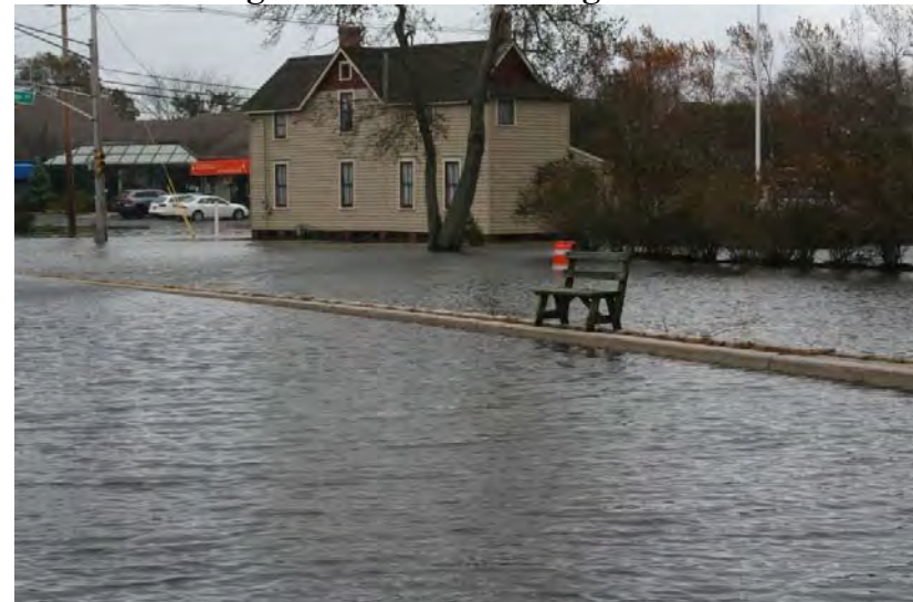
Figure 2: Flooded Borough Street
