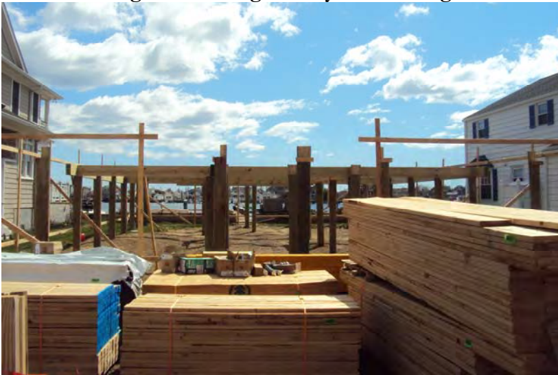
Figure 11: Pilings Ready for Framing
